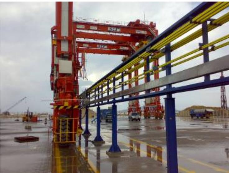
*BU: Conductor bar systems supply electrical power using a current collector trolley that moves back and forth on a steel structure.*
