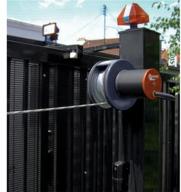
Slip ring assembly in gate locking system
