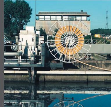
Motorized cable reel on a linear scraper bridge
