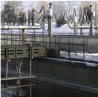
Main power supply of a longitudinal scraper bridge in a waste water treatment plant
